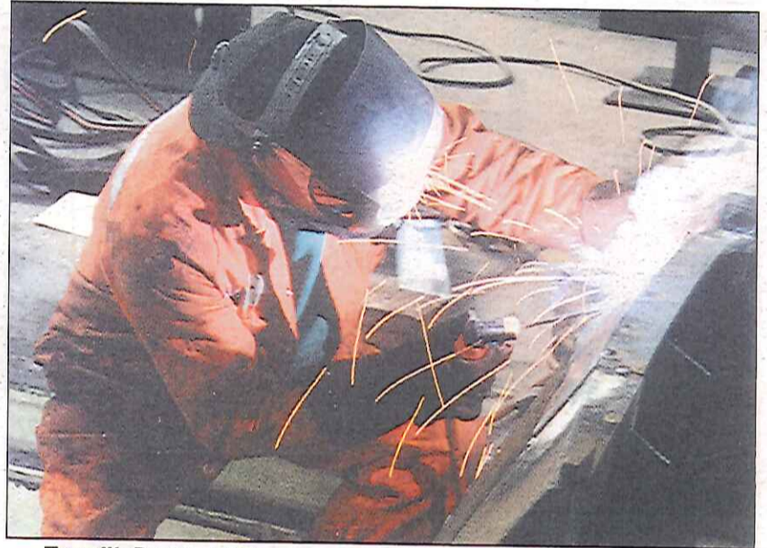
Tasrail's Paul Ralph does some welding repairs to a DC locomotive.
